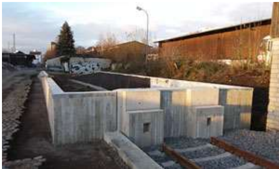
FIGURE 11: HEAD RAMP (UNDER CONSTRUCTION IN BONN-BEUEL FOR LOADING CIRCUS TRAINS) 2
