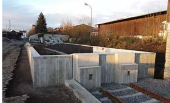
Figure 10: Head ramp (under construction in Bonn-Beuel for loading circus trains) 2
