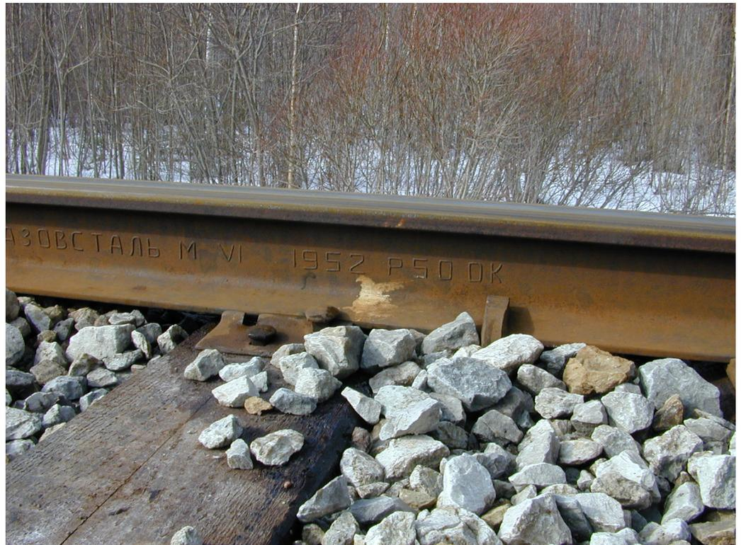
Figure 5.5 Jointed track, wear between the rails. The Pärnu line
