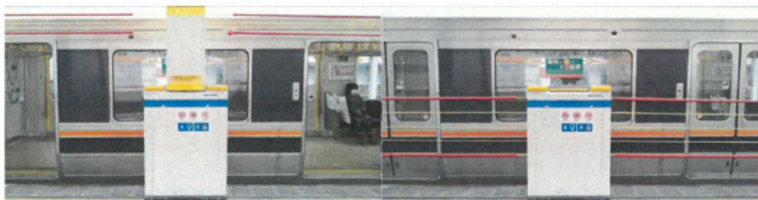
Figure 13: Platform fences with wires in Japan (Sakurajima Station) – side view
