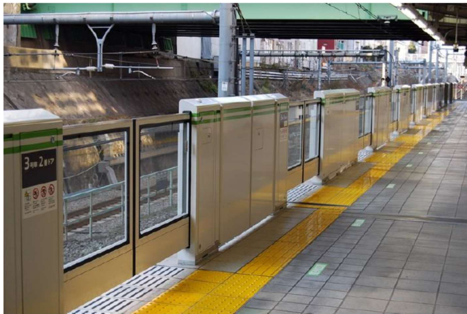
Figure 12: Platform fences with automatic gates in Japan (Meguro Station)
