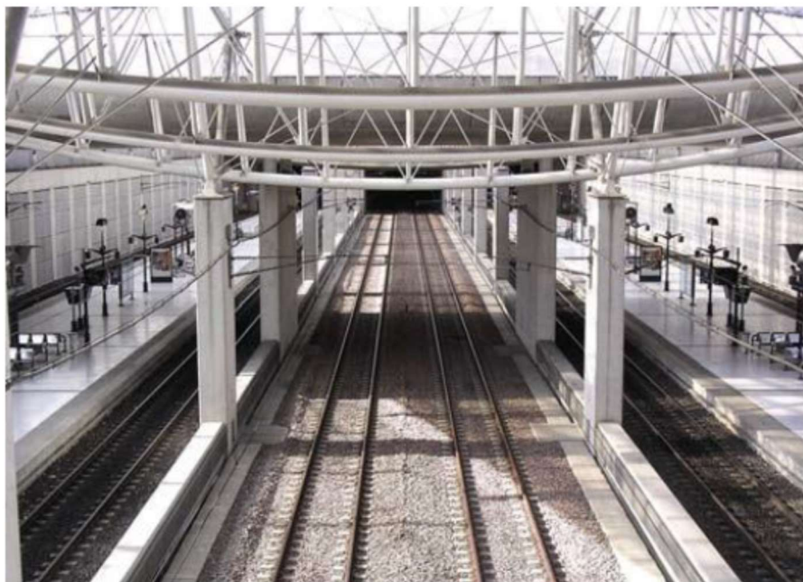
Figure 6: French high speed station (St. Raphael) with separate through tracks and passive barriers
