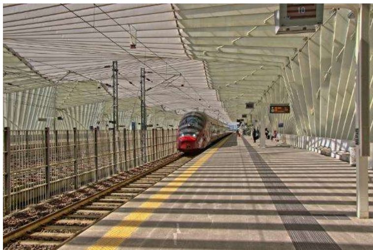
Figure 3: Example of passing track with fixed fences in Italy (Reggio Emilia station)
