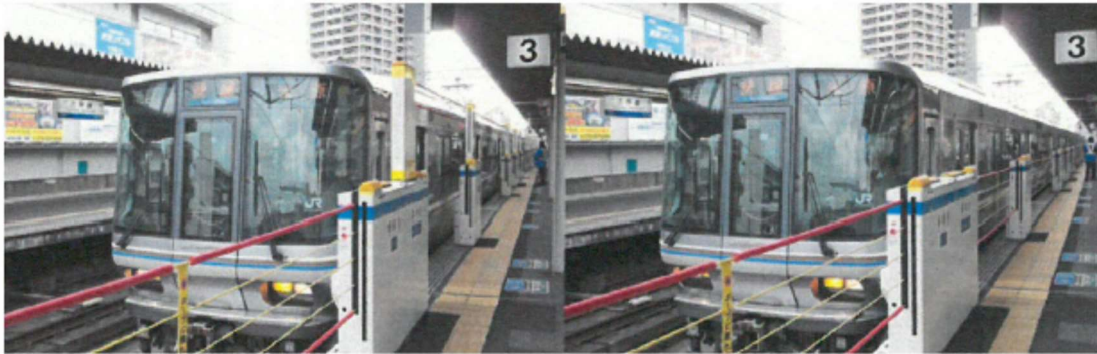
Figure 14: Platform fences with wires in Japan (Sakurajima Station) – front view
